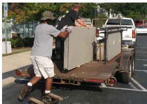
Crew loads panels on trailer
