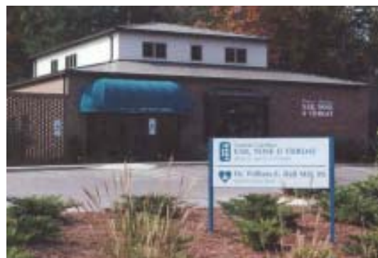
1915 KM Wicker Drive Sanford, NC 27330
