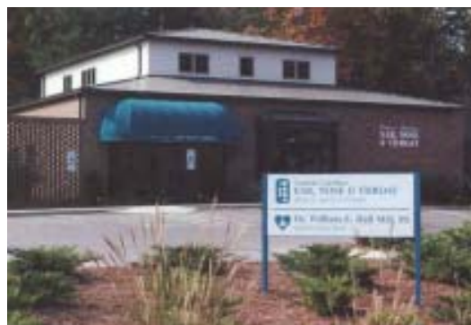
1915 KM Wicker Drive Sanford, NC 27330
